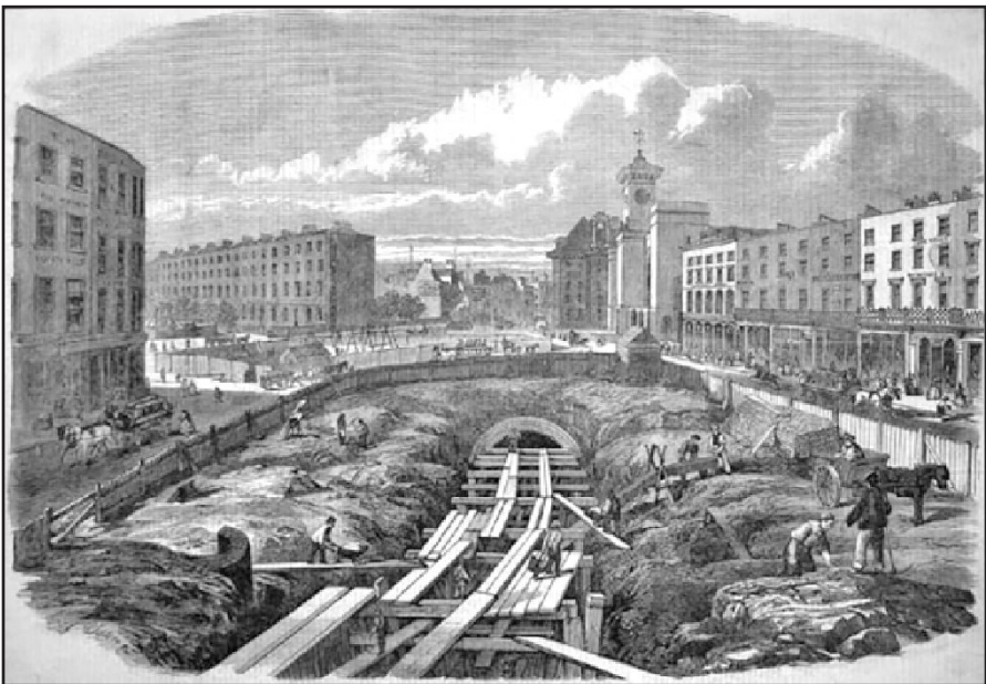
Fig. 1. Cut and cover construction, 1861. wikipedia.com
